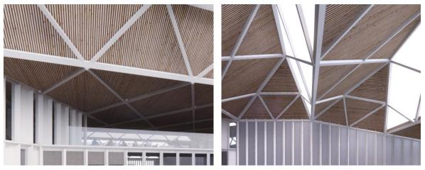
Figure 48. Wooden slats ceiling on main entrance area (left) and opaque gables (right)
