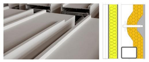
Figure 60. Mockup of GRC façade. Section detail of GRC wall
